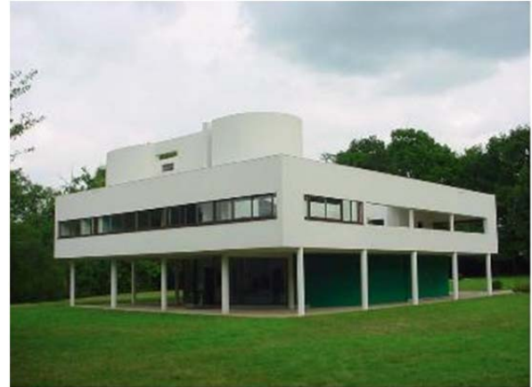
Fig. 8: Exterior view of Villa Sayoye, Poissy, France
